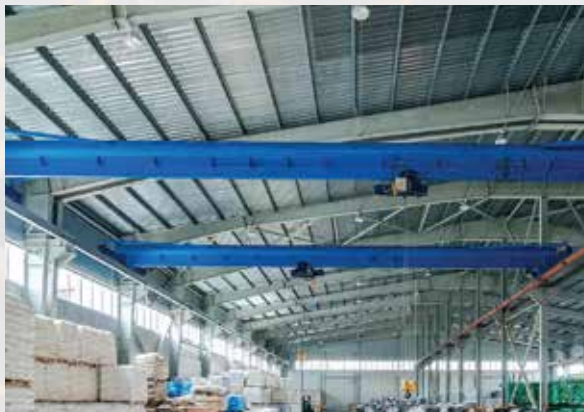
Under Deck Insulation
